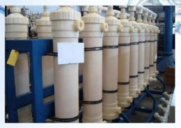
**Ultrafiltration (UF)** is a membrane filtration process similar to Reverse Osmosis, using hydrostatic pressure to force water through a semi-permeable membrane. The pore size of the ultrafiltration membrane is usually 103 - 106 Daltons. Ultrafiltration (UF) is a pressure-driven barrier to suspended solids, bacteria, viruses, endotoxins and other pathogens to produce water with very high purity and low silt density.
